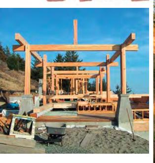
from kiln-dried finger-jointed 2x Douglas fir (photo below left). Glulams are remarkably strong and stable, and lend themselves to big cantilevers—something we took advantage of at the entry to the house (photo below right). The bolted steel-plate connectors that we used to join beams to posts are so strong that we could do away with angled braces.
